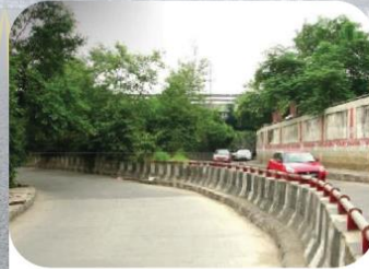
DEFENCE COLONY UNDERPASS
